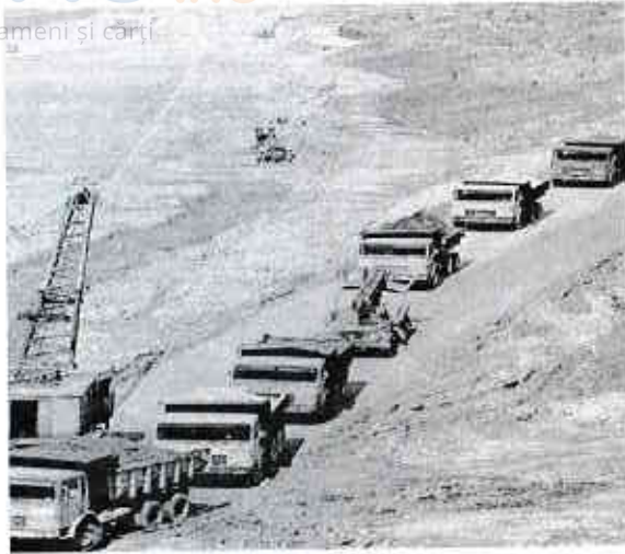
Danube Channel - Black Sea - construction site
